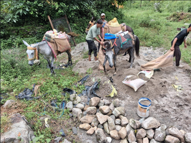
Mule caravans transporting construction materials to remote Himalayan site, August 2026
