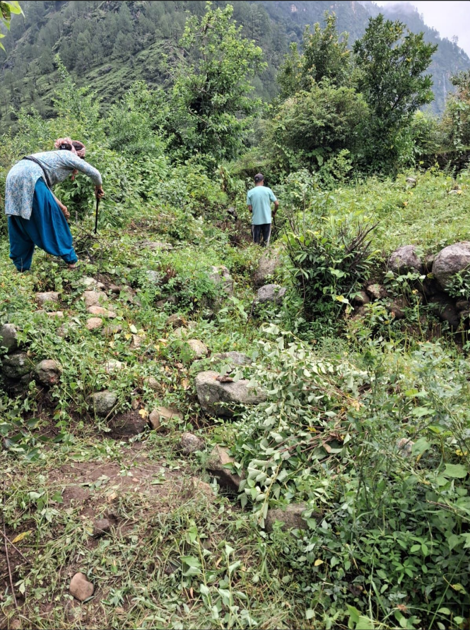
Material transport and site preparation, Mandal Valley, July 2026
